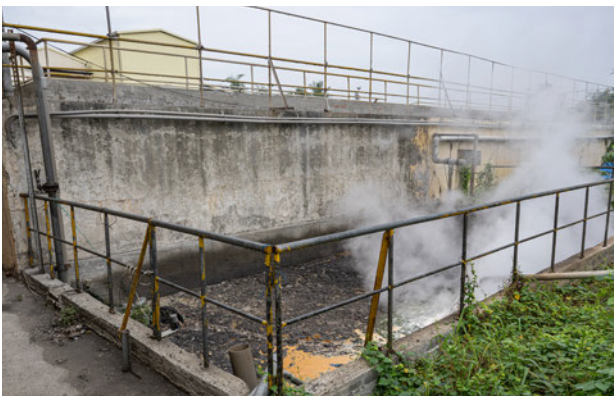
Wastewater discharge area at a textile factory supplying lululemon in Taiwan
