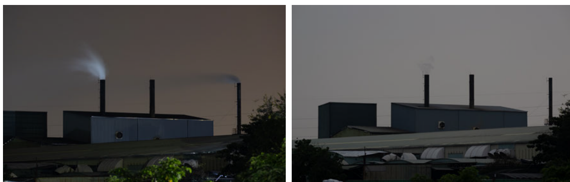
Smoke from chimneys during day time; [right] and night [left] at a textile factory supplying lululemon in Taiwan.
