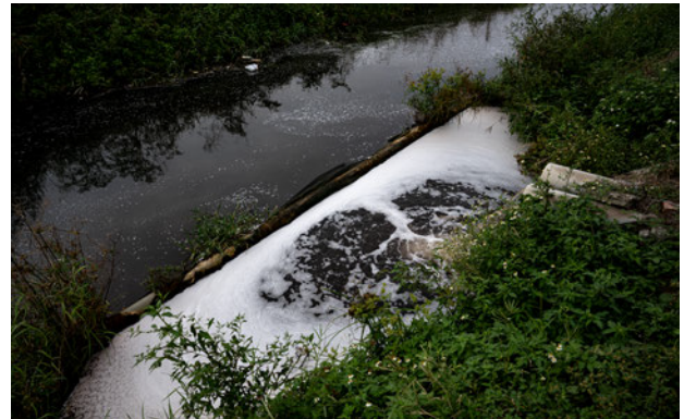
Wastewater discharge area at a textile factory supplying lululemon in Taiwan
